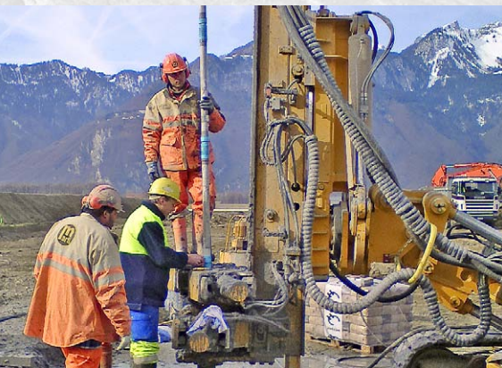
Installation of measuring tube in borehole
