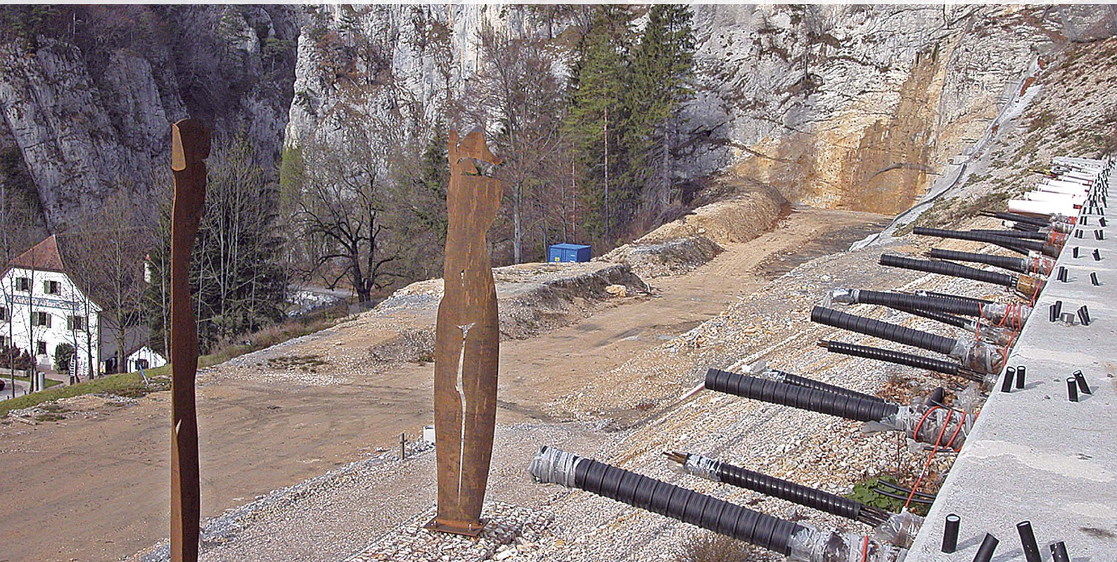
Transjura Motorway A16, construction of the section Roches-Moutier, Canton Berne. Trivec measurements in a pile wall
