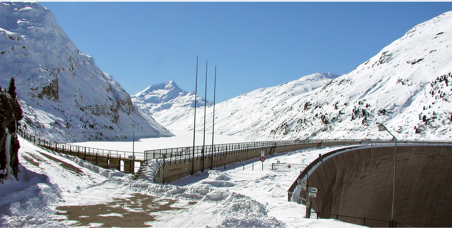
Val di Lei Dam, Sliding Micrometer measurements in the dam foundation
