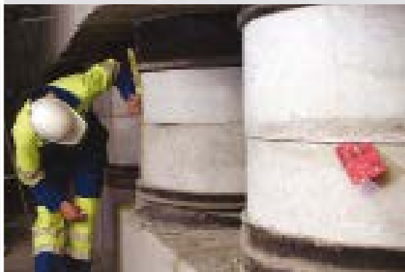
hiDCon foundation elements in the Chienberg tunnel
