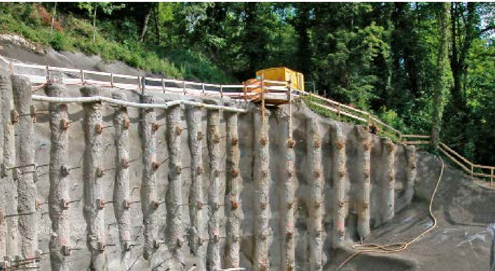
Aarburg bypass, Canton Aargau: Monitoring of excavations
